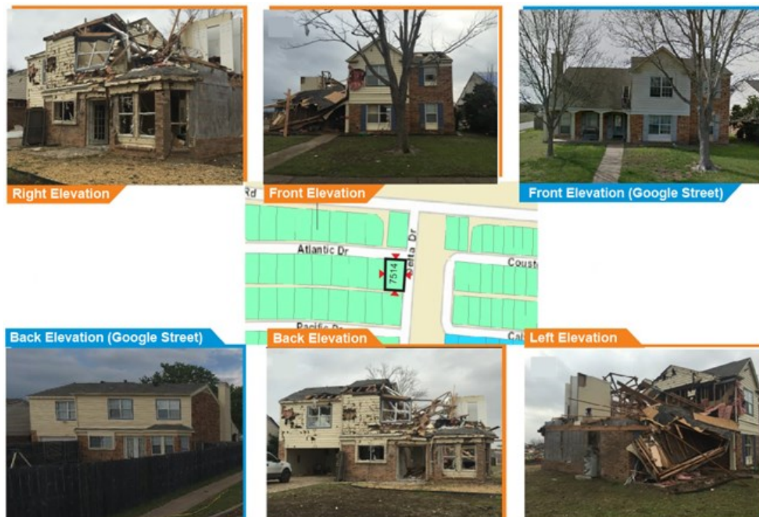
Figure 3. Photographs of Elevations of a Damaged House (7514, Atlantic Drive Rowlett, TX) and comparison with Pre-Tornado Image (from Google StreetView)
