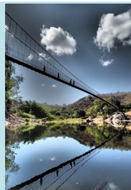
Paso Real Footbridge, Nicaragua
