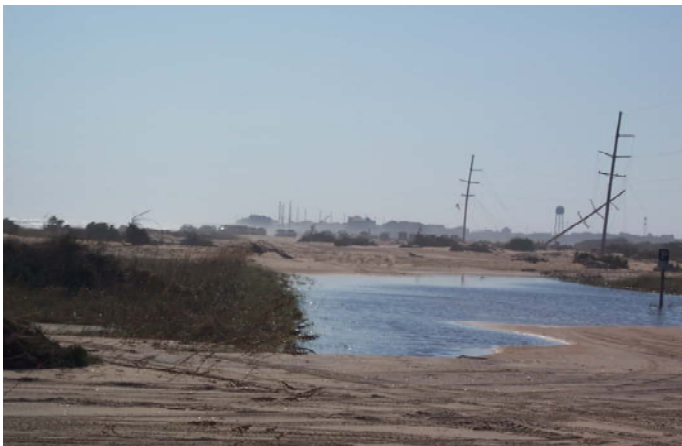
Figure 5. Area Around Outer Banks, Near Tower Site
