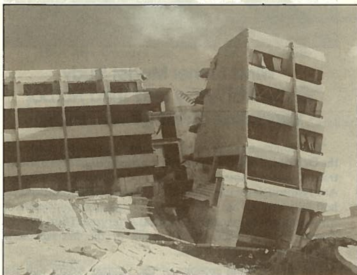
Storm Surge and Wave Action Damage to Hotel Buildings Sited Near Water at Isla Cancun
