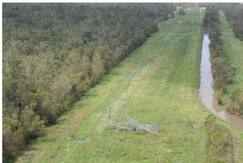
Multiple failures of high tension lines devastate the power grid.
