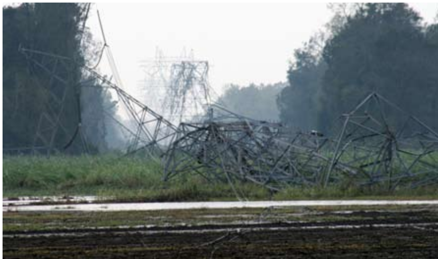
Multiple transmission tower failure.
