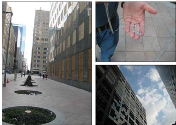
Figure 5: Uprooted Trees between Buildings (left), Glass Fragment from Chase Tower (top right), and Window Damage to Parking Garage (bottom right). (Photos by ABS Consulting)
