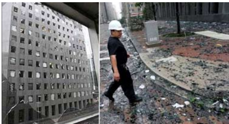
Figure 2: Next-Morning Damage Photos
