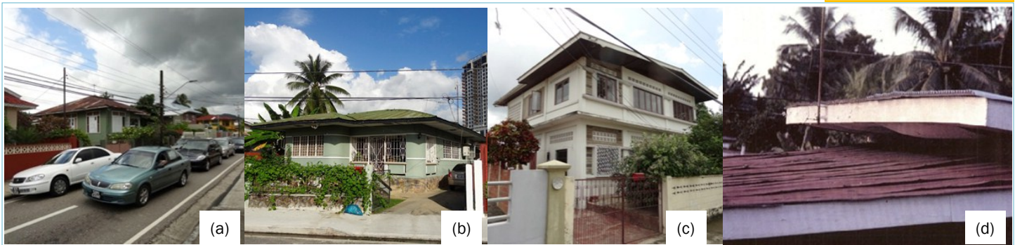
Figure 2. (a) Typical residential neighborhood in Port of Spain, Trinidad. (b) Single- and (c) two-story modern concrete masonry block homes with large eaves extending outwards on all sides. (d) A 1.2 m (4 ft) wide cantilever roof overhang at the ridge of a double-lean-to roof, northwest Trinidad, (Photos by David O. Prevatt)
